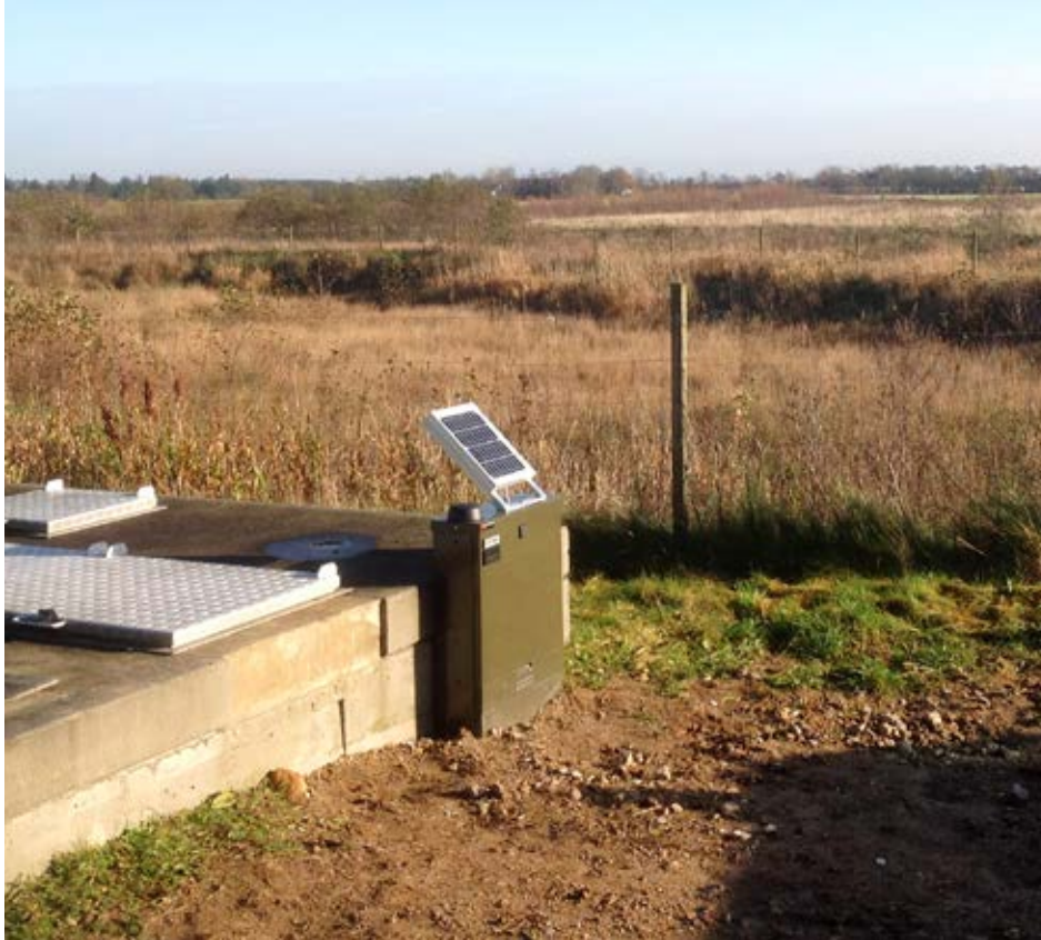
As sewer overflows are often very remote, and rarely established with a main power source – the complete system is battery powered, with the possibility of direct connection to a small solar panel, for permanent operation.
