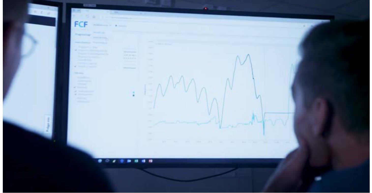
Control panel at Rya wastewater treatment plant in Göteborg, Sweden
